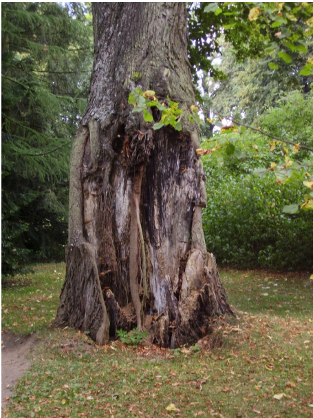
Fig. 18: Damaged tree base
