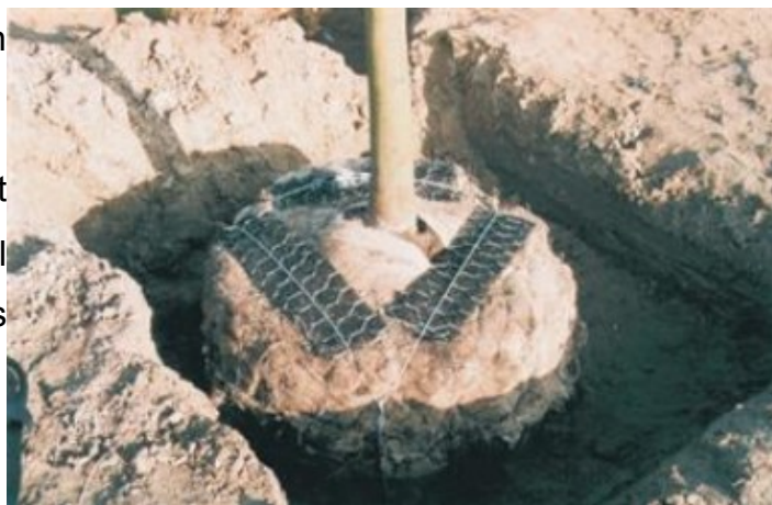
Fig. 25: Underground anchoring
