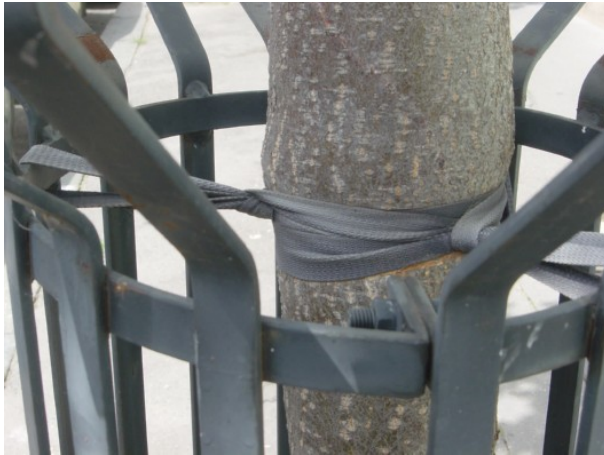
Fig. 24: Wrong anchoring, must be removed.
