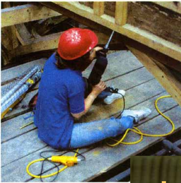
FIG 16 Coring a large tiebeam in the G Windsor Castle (English Heritage Centre)
